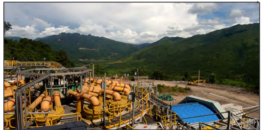
Typical Alumina HydroCyclone system
