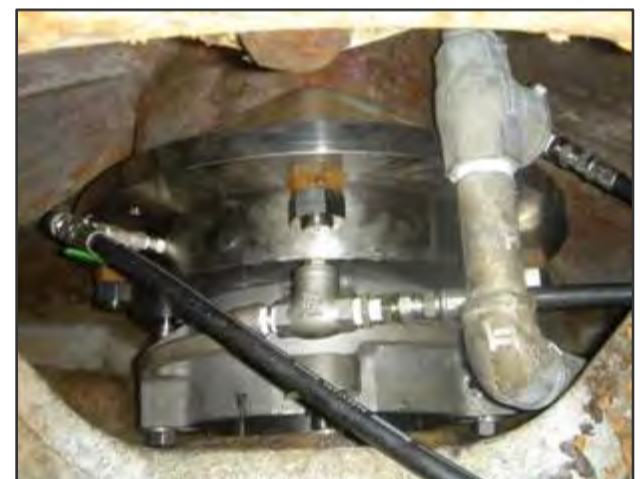
Installed Chesterton Engineered Solution
